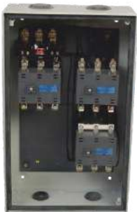
Interior View of ML SASD
