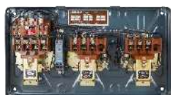
Interior View of MK2 FASD
