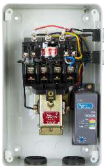
Interior View of MK1.i
