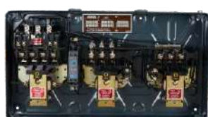
Interior View of MK1 FASD
